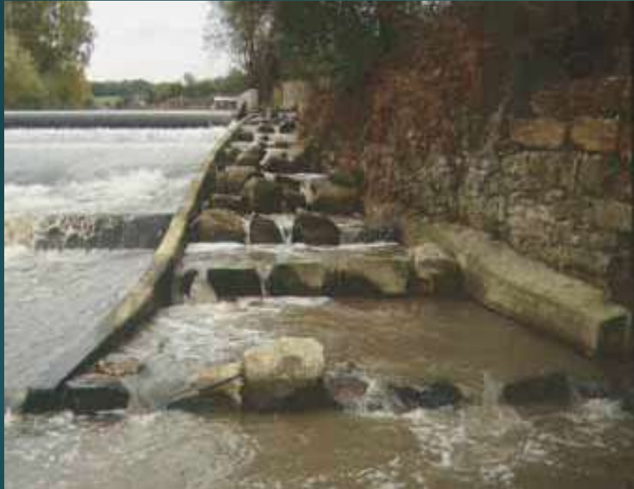
Uhingen/Fils rough-channel pool pass View from tailwater end.
